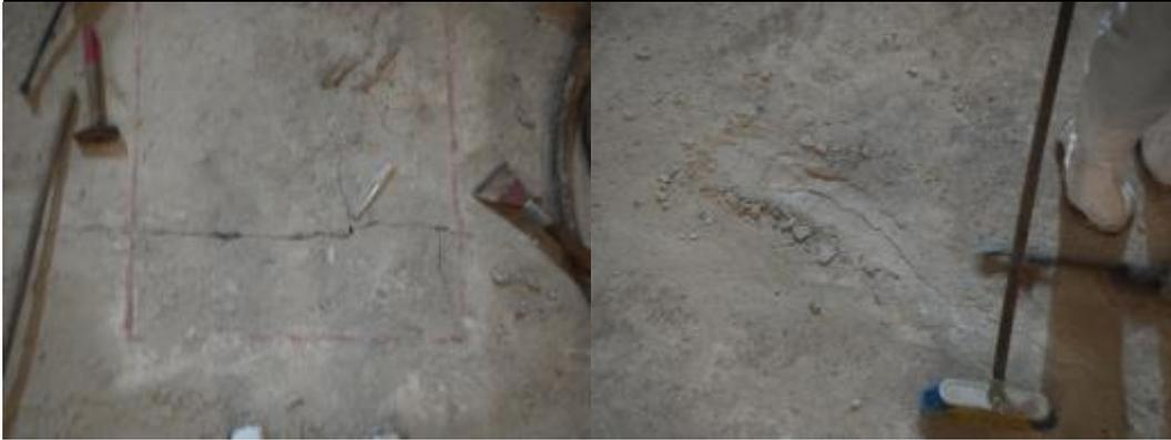
**Figure 8.1 Large cracks in site floors (warehouse 4)**
